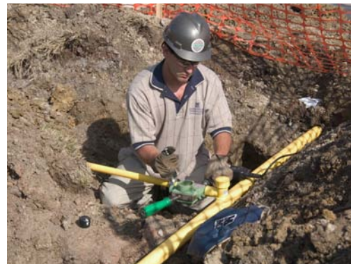
The new McElroy Socket Tooling Kits offer contractors great value in a specially designed tool box (left). A fusion technician socket fuses a service connection (above).
